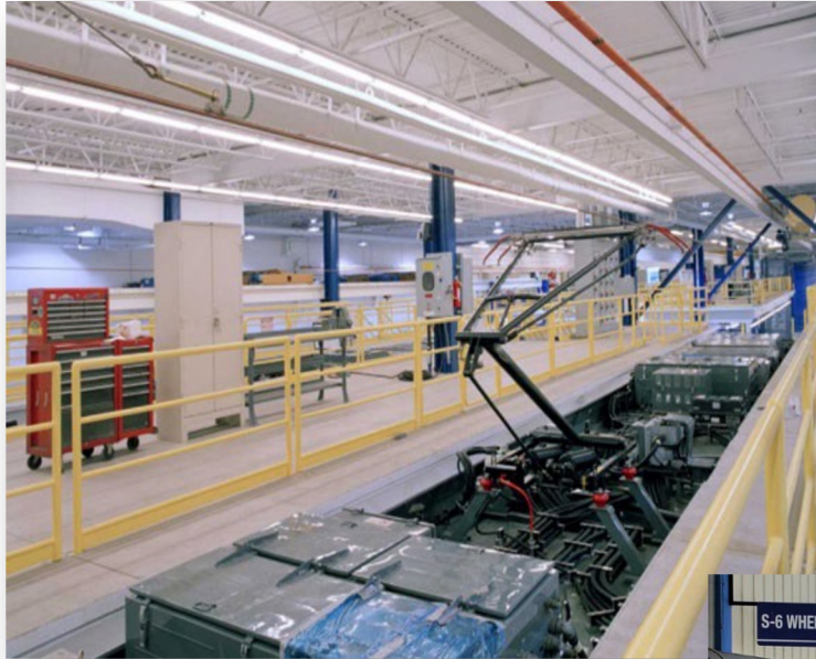
Increased Roof Access
