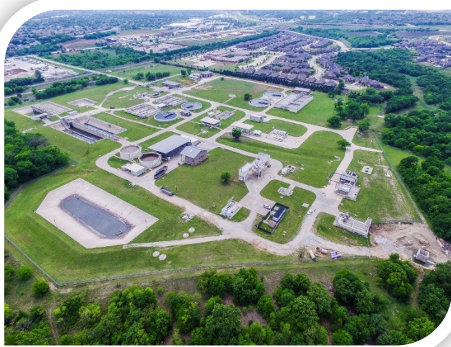
Denton Creek Regional Wastewater System (11.5 MGD; 13,000 WTY)
