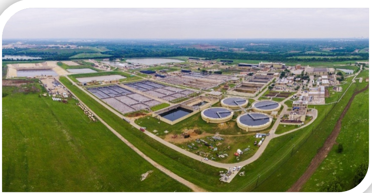
Central Regional Wastewater System (189 MGD; 273,020 WTY)
