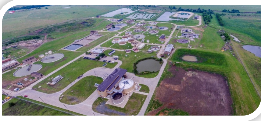
Ten Mile Creek Regional Wastewater System (24 MGD; 13,000 WTY)
