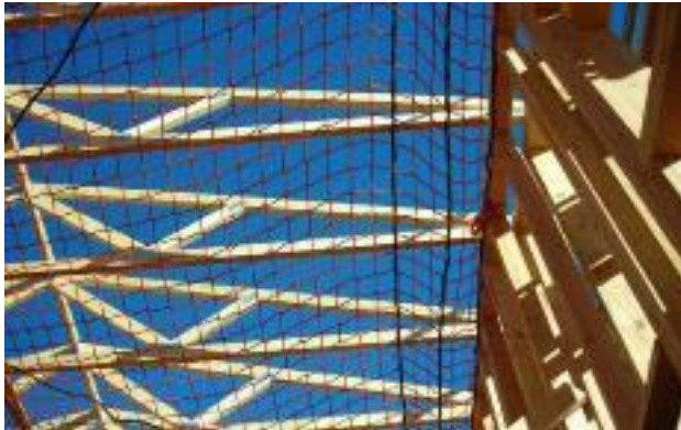
Safety Net in Residential Construction
