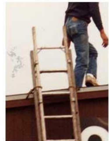
Ladder secured to roof.
