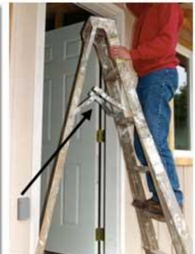
Danger! The spreader isn't fully open (WAC 296-876-40050).
