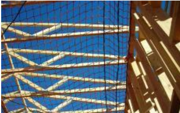
Safety Net in Residential Construction
